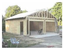
The above type buildings require a standard 16"wide x 12"deep x 8" thick concrete poured footing, or a monolithic type "turn down" slab /footing combination as shown below...
